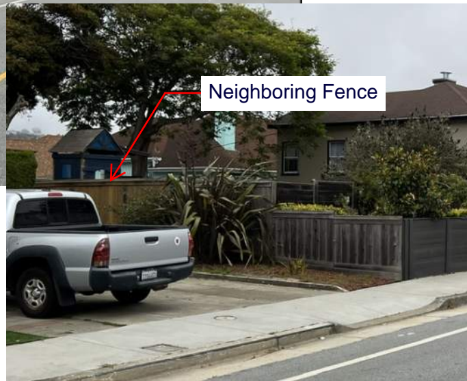
Bottom Photo: captured on 7/8/2024 along Holloway Ave. near Ashton Ave. intersection. Unauthorized fence remained encroaching into the public right-of-way own by County of San Francisco.
