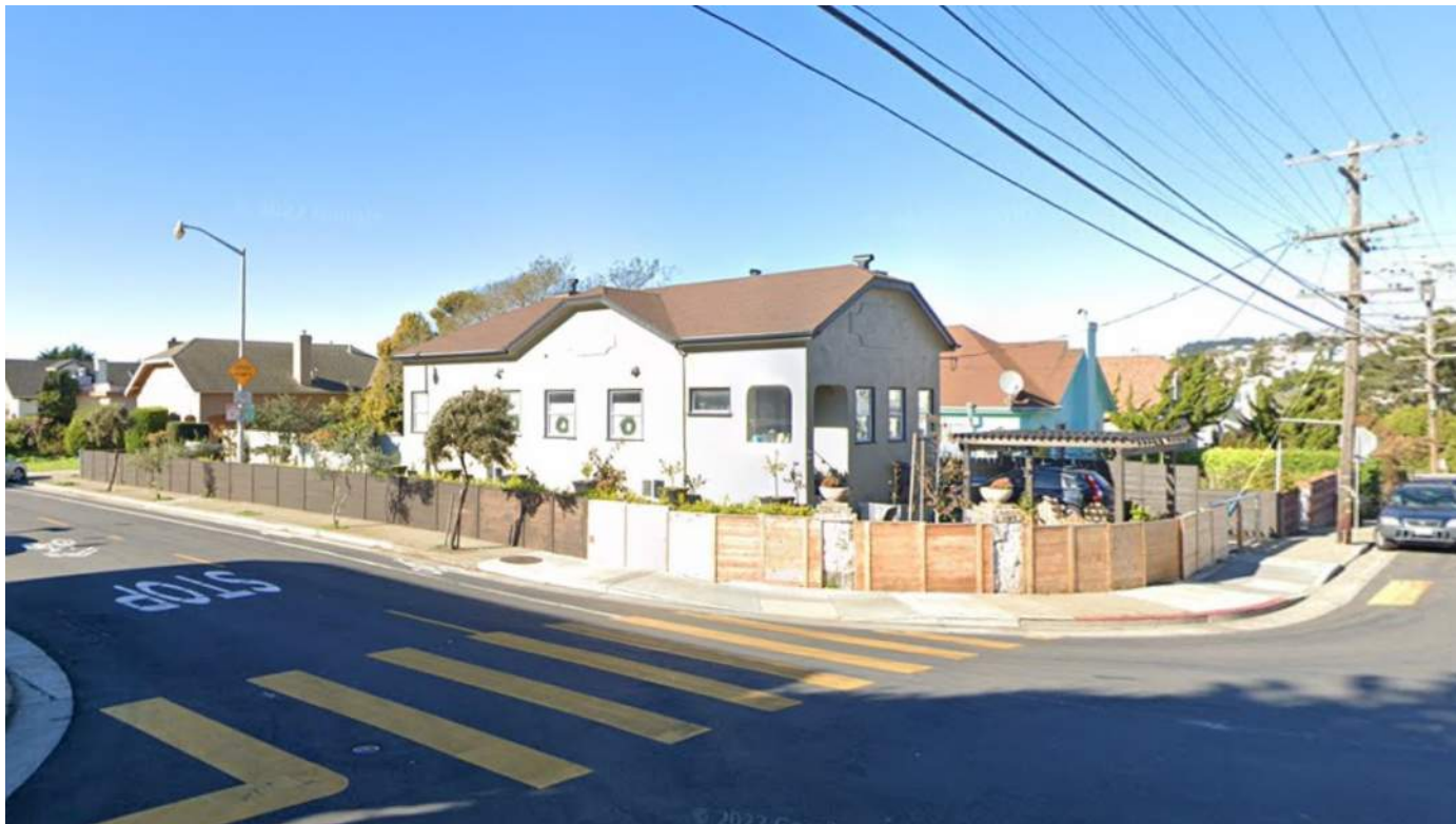
Bottom Photo: Captured in 2017 (Source - Google Map) Observed unauthorized wooden fence erecting surrounding the frontage of premises along Ashton Ave and Holloway Ave.
