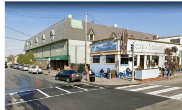
SLOAT & 45TH AVE- SOUTH WEST
