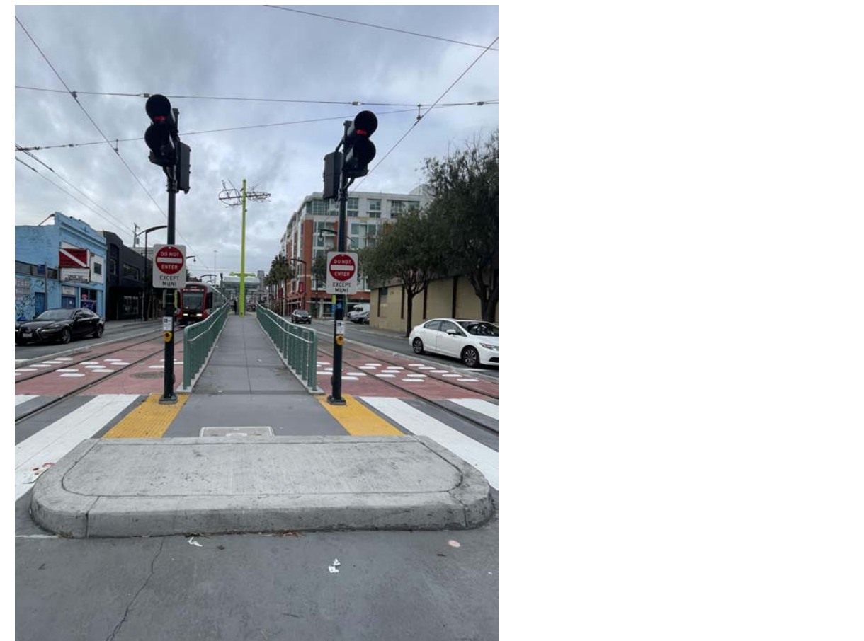
12. 4TH AND BRANNAN STREET STATION NORTH CROSSWALK
