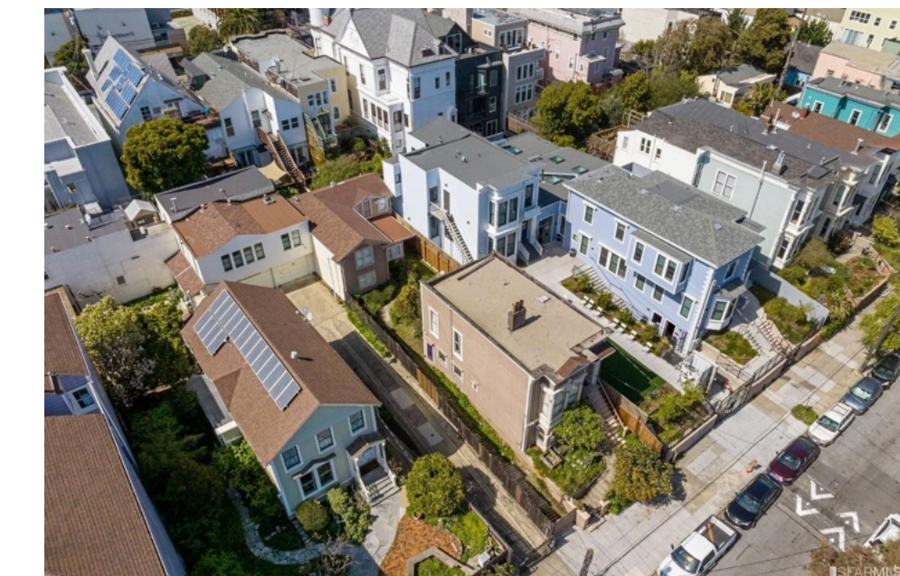
AERIAL VIEW SOUTH FACADE
