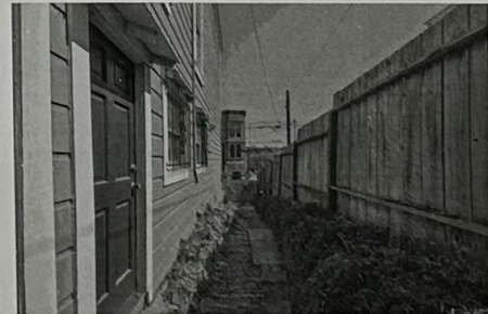
SOUTH FACADE DETAIL
