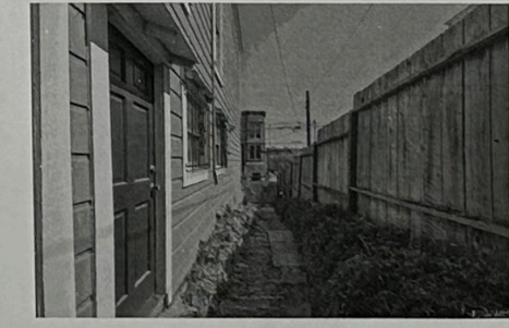
SOUTH FACADE DETAIL
