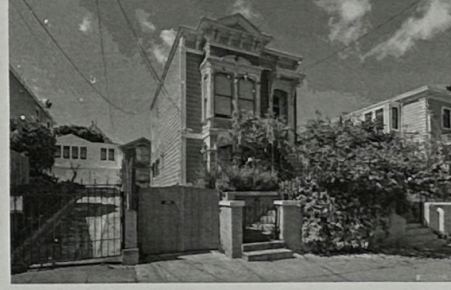
FRONT FACADE VIEW
