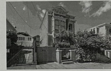
FRONT FACADE VIEW
