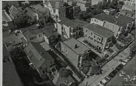
AERIAL VIEW SOUTH FACADE
