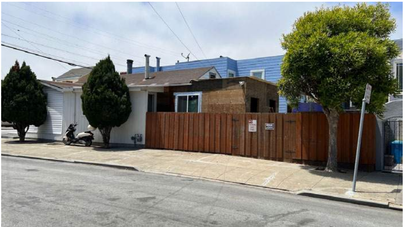
Rear addition remains unprotected from weather and fire.
