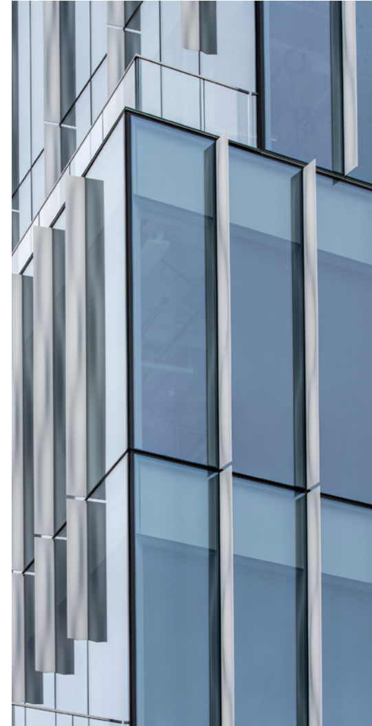
GLAZING WITH LOW-E COATING LEVELS 5-7
