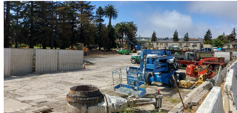
2 SITE PIT FROM REMAINING OLD BUILDING
