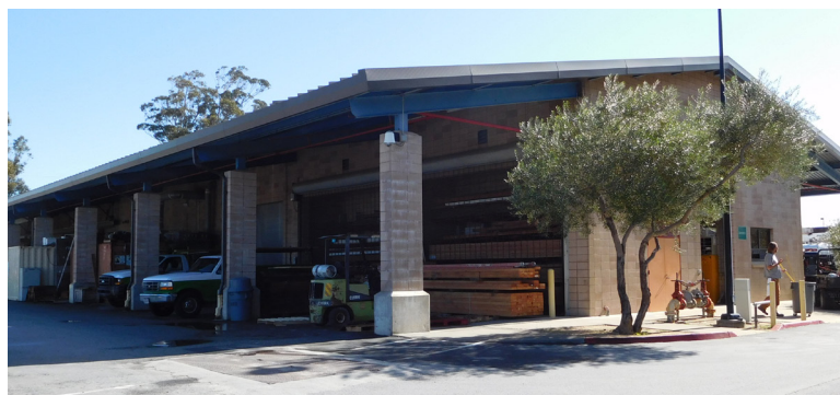
7 NORTH SHOP BUILDING
