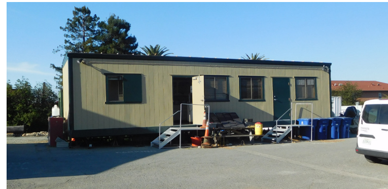
6 TEMPORARY TRAILERS TO HOUSE GROWING STAFFING NEEDS
