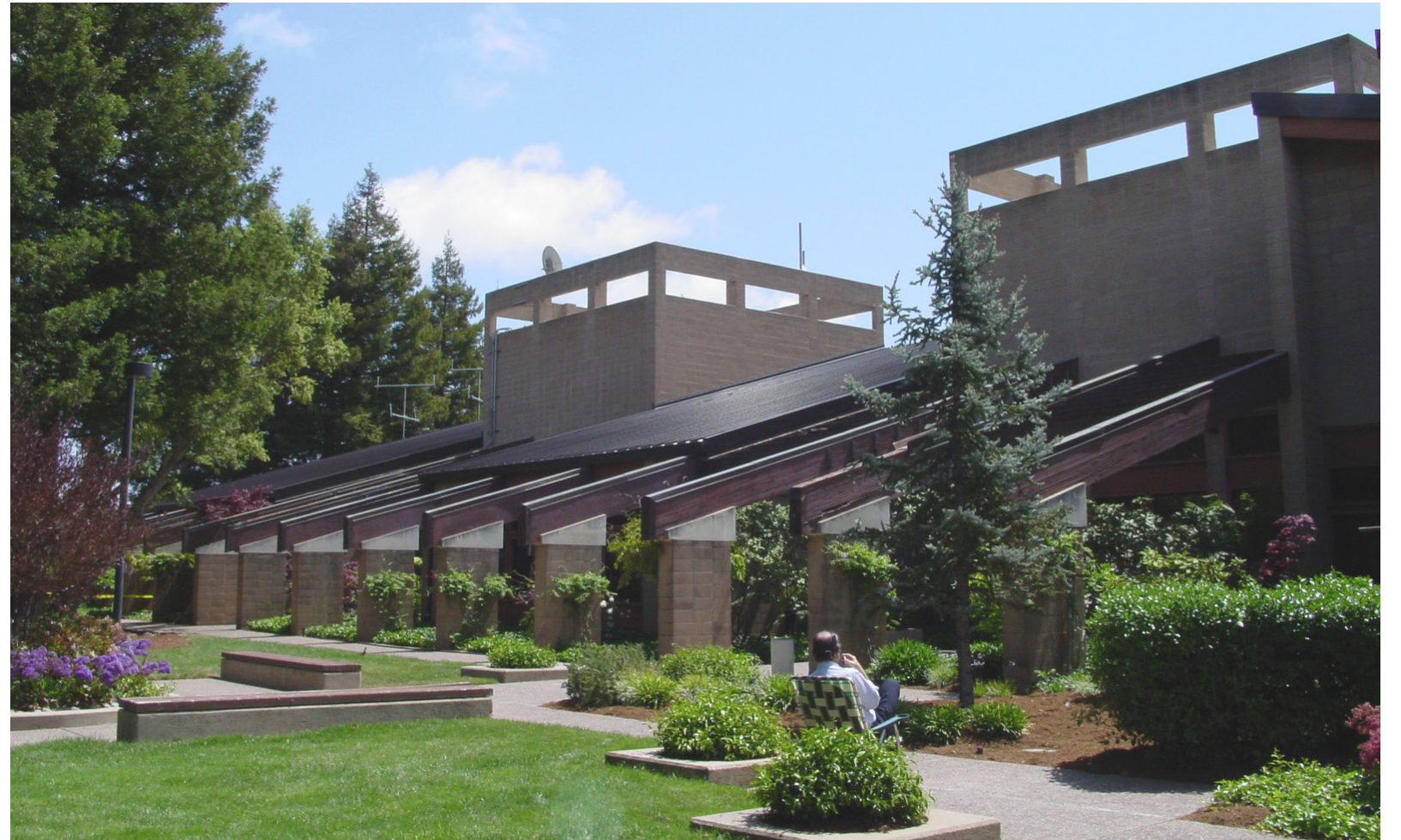
EXISTING ADMINISTRATION BUILDING TOWARDS LOBBY ENTRY
