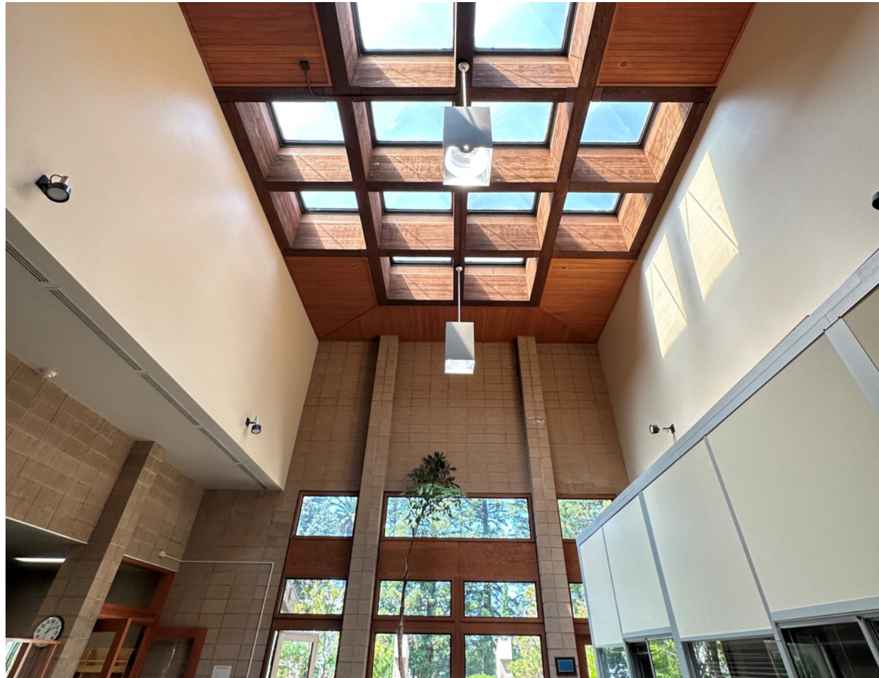
EXISTING ADMINISTRATION BUILDING DOUBLE HEIGHT LOBBY
