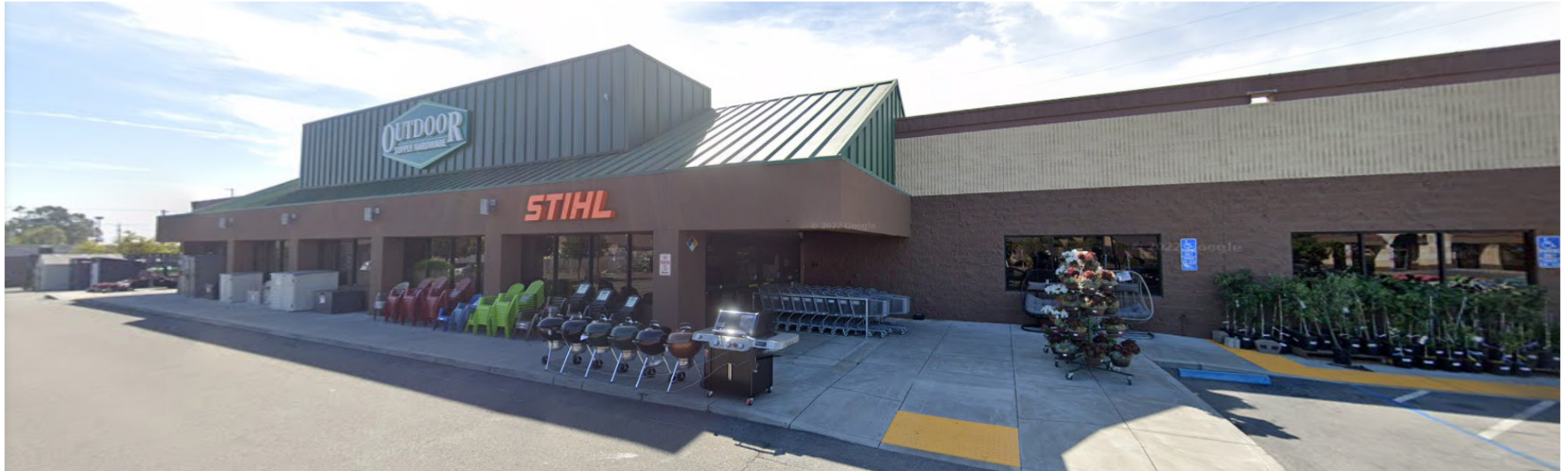
EXISTING OSH RETAIL MAIN ENTRY
