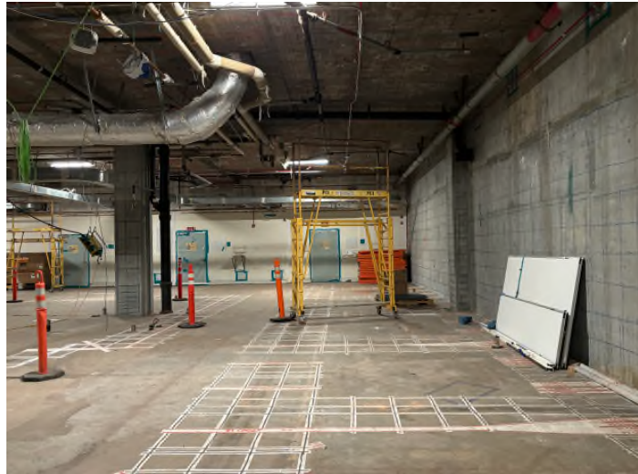
Floor Scanning – Locating Rebar and Post Tension (PT)
