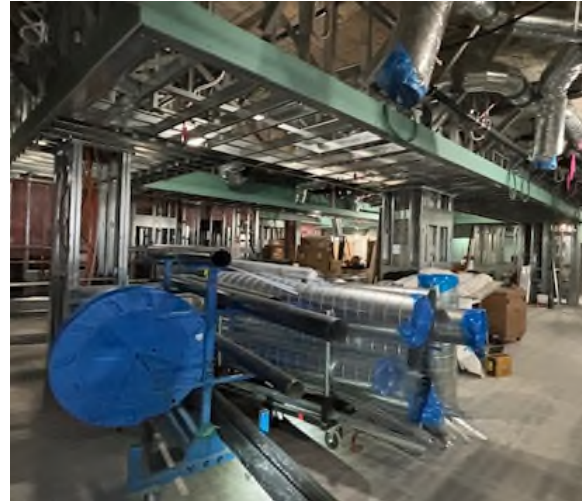
Nurse Station / Treatment Bay
