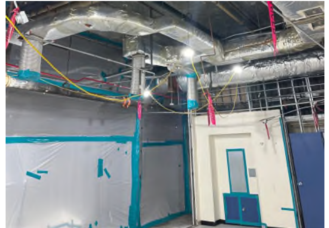
Haz Mat Abatement Containment at Bedshop Area, Basement Level
