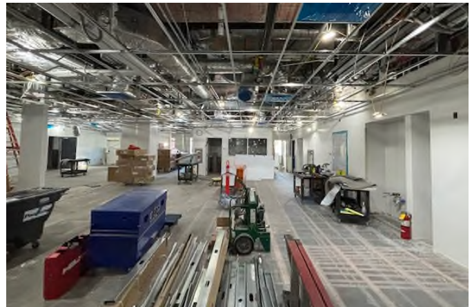
Office Space Area
