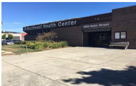
Existing SE Health Center
