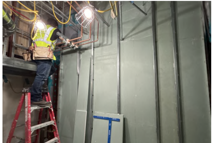
Sheetrock Installation in Waste Holding
