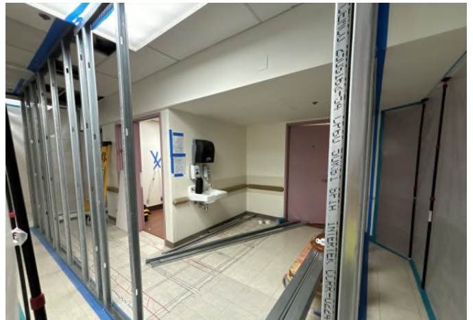
Temp Construction Barrier Ward 3C Restroom
