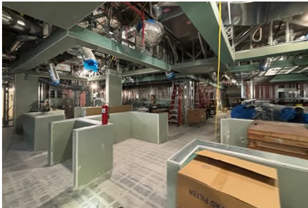
Nurse Station / Treatment Bay Sheetrock Installation
