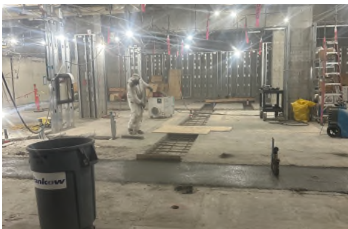
Plumbing Trenching – Concrete Slab Reinforcing Steel Installation at Floor Slab (Before)
