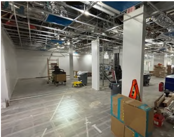
Future Track Equipment Area
