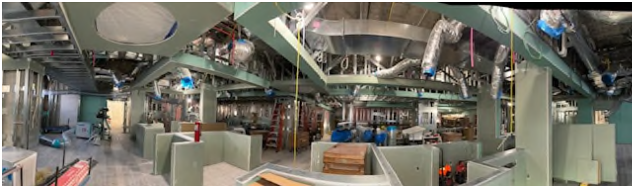
Nurse Station/Treatment Bay Panoramic View
