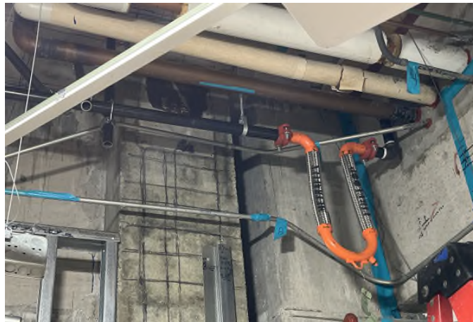
L3 Seismic Joint Flexible Connection_
