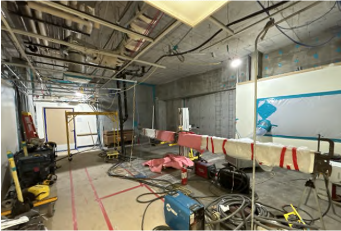
L3 Seismic Joint Structural Steel Beam Prep
