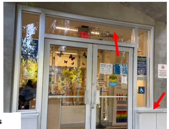
Completed Caulking Scopes
