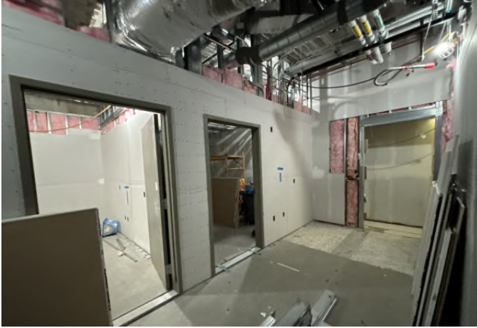
Sheetrock Installation and HVAC in Urology
