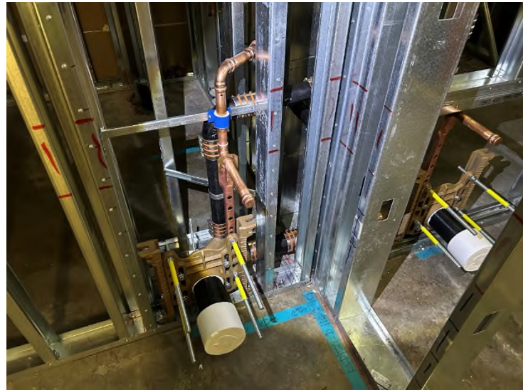
Shower room water closet installation
