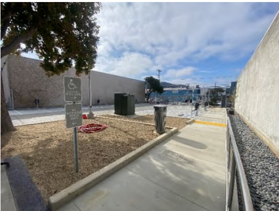
Rear Parking Lot
