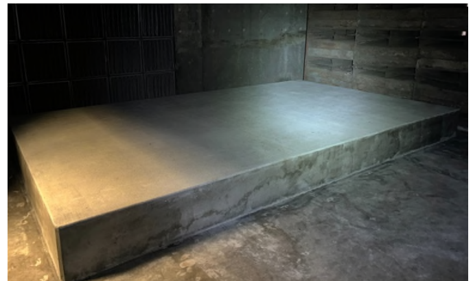
New Air handling Unit (AHU) Concrete Pad at Basement Level
