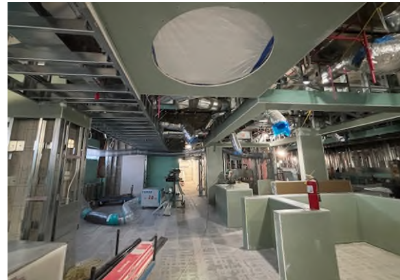
Nurse Station / Treatment Bay Sheetrock Installation
