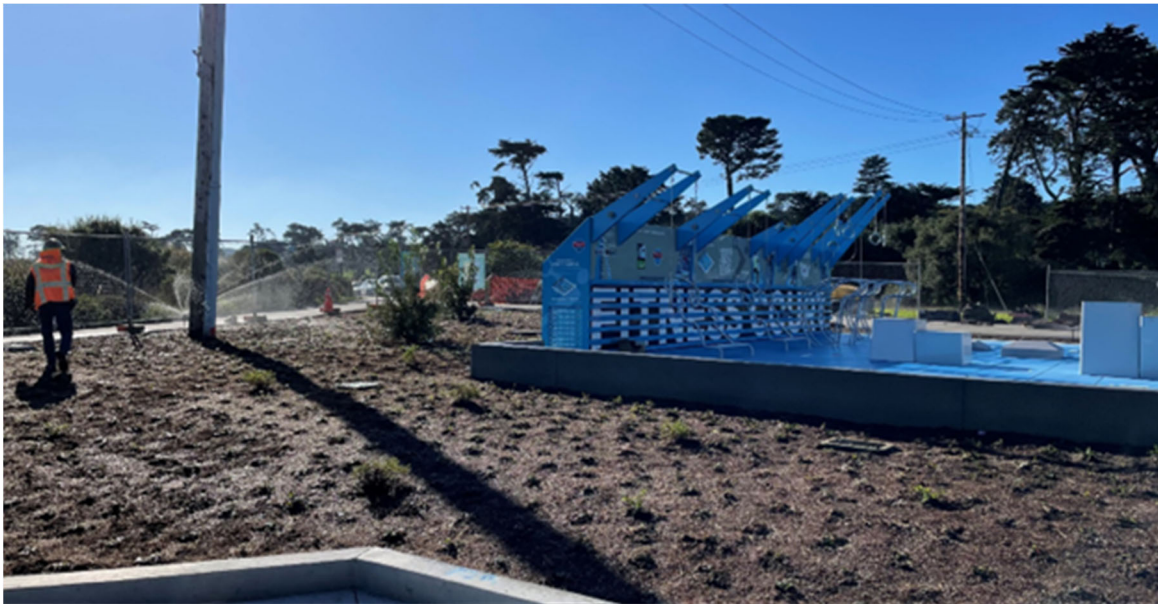
Lake Merced Construction (May 2024)
