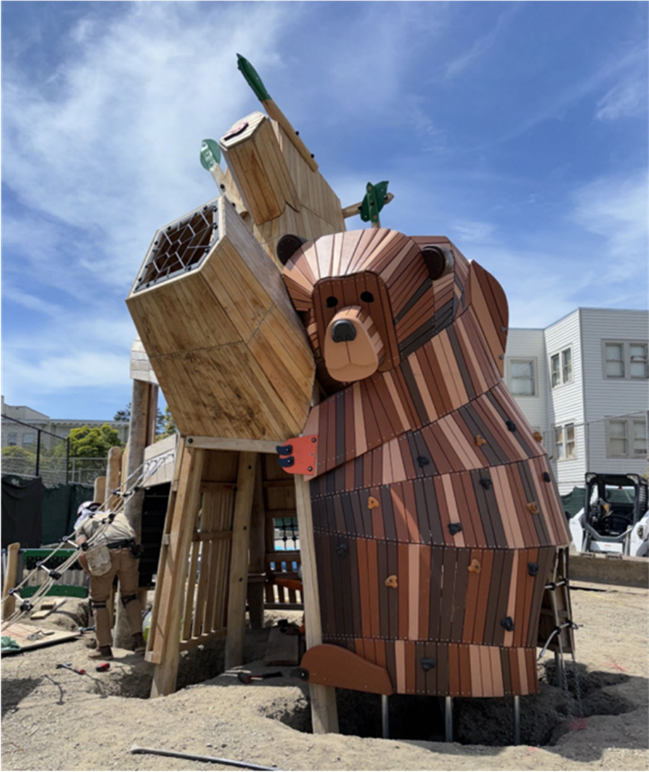
Richmond Playground – Construction Spring 2024
