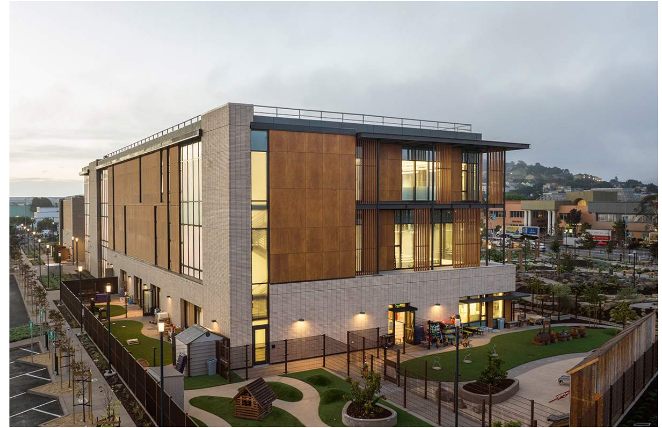
Community Center by BOA - near site
