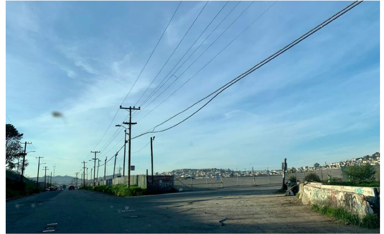
VIEW LOOKING NORTHWEST ALONG CARROLL FROM GRIFFITH
