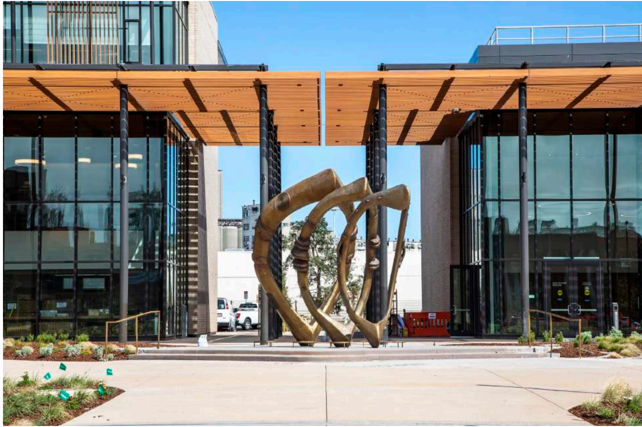
Community Center by BOA - near site
