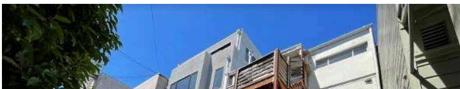
45-49 Bernard Rear of Building
