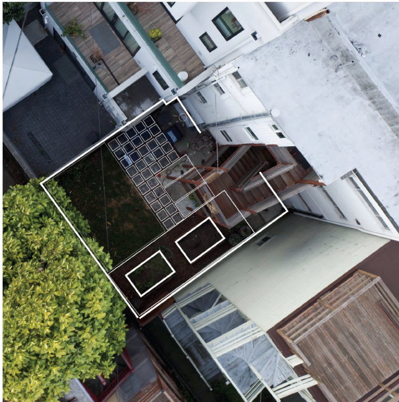
Figure 1. The Chinese courtyard outlined in white at 45 Bernard Street.
