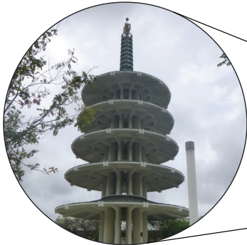
PEACE PAGODA (structural upgrade)
