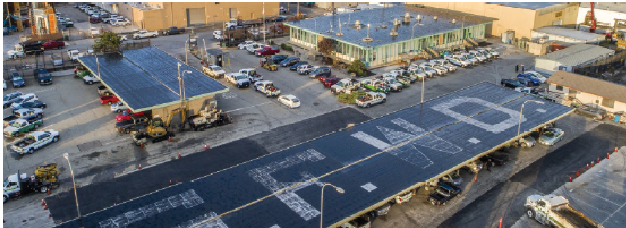
Existing site mixes pedestrian and vehicular paths across the sprawling campus.
