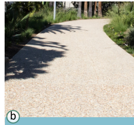
b Exposed aggregate concrete (2 depths of exposure for hierarchy)
