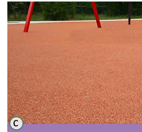
c PIP safety surface at fitness
