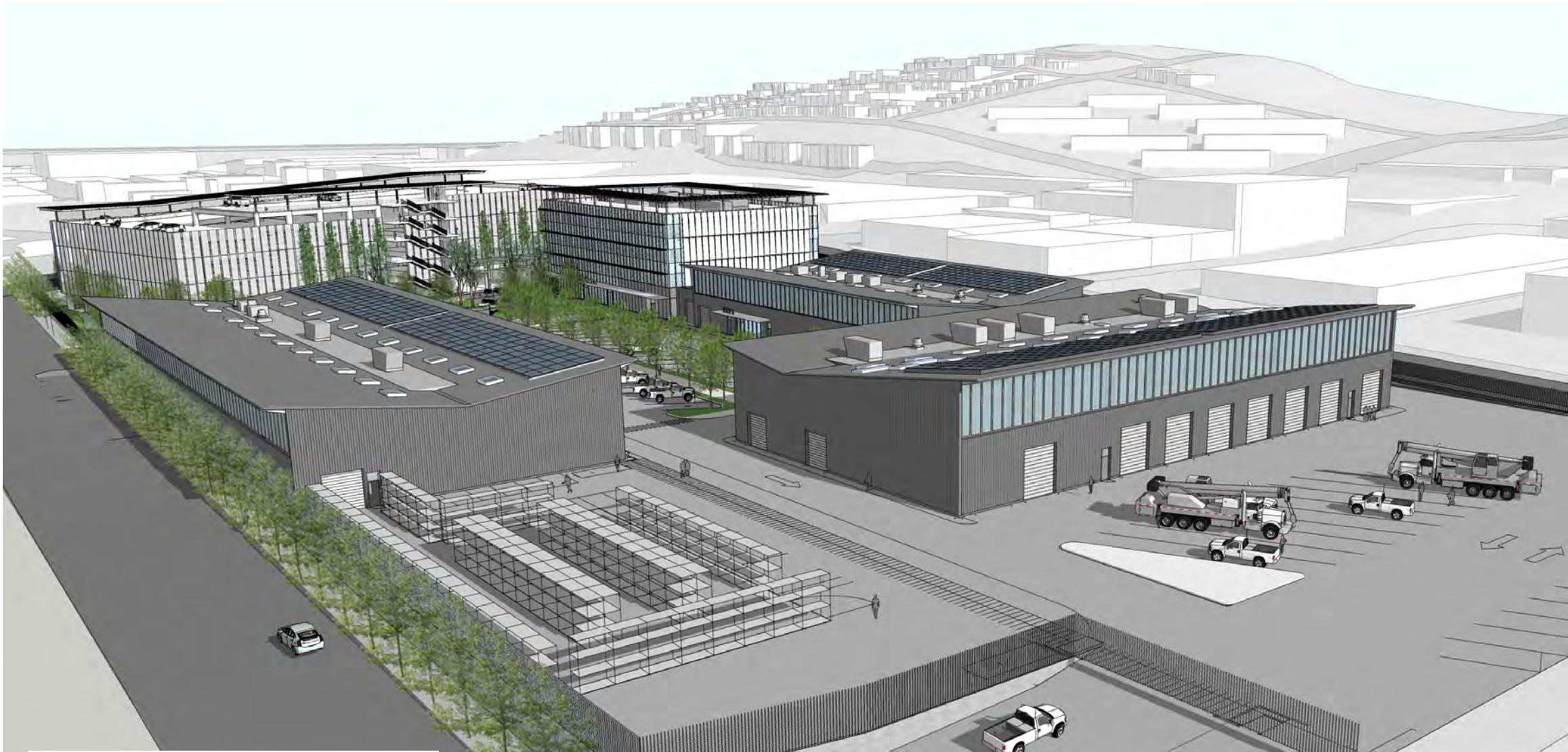
CAMPUS VIEW | LOOKING NORTHWEST TOWARDS POTRERO HILL
