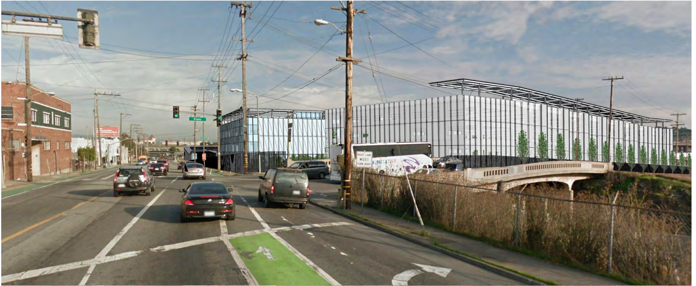
CAMPUS VIEW | LOOKING EAST AT CESAR CHAVEZ/EVANS INTERSECTION
