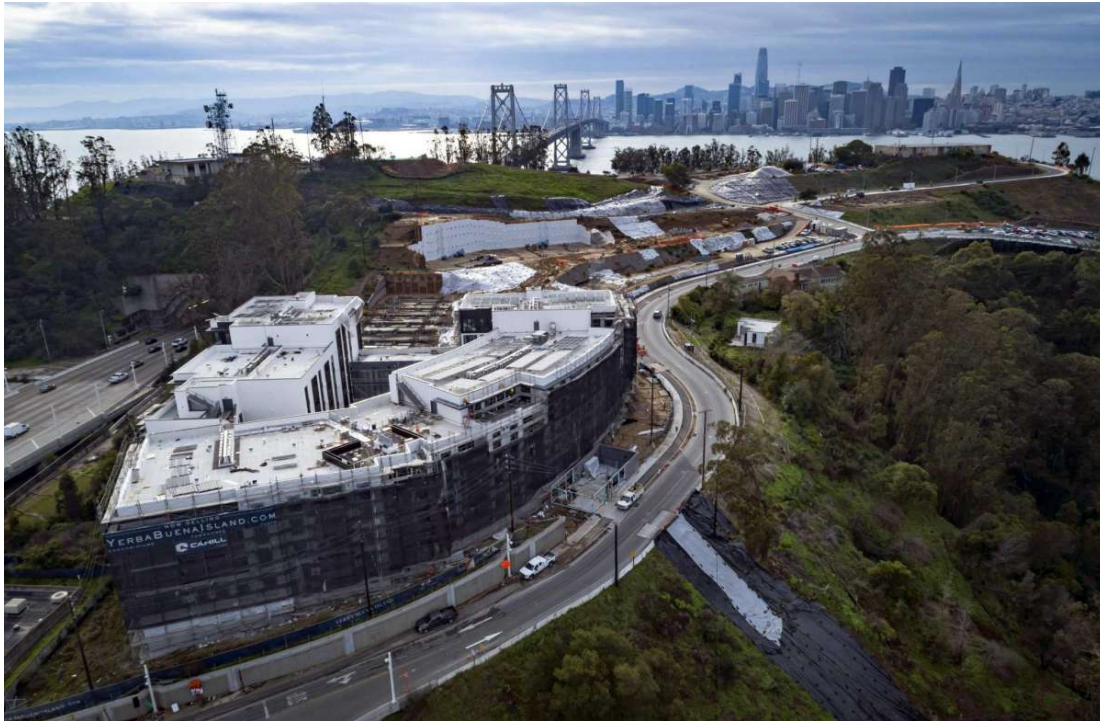
The new Bristol Condominiums on Yerba Buena Island in San Francisco.
